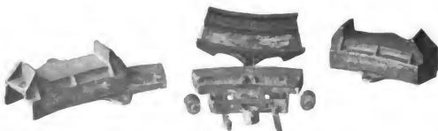
Figs. 4519-4521. Susemihl Roller Side Bearing American Steel Foundries.
